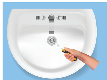
59-rasm. Sifonni yechib olish.
