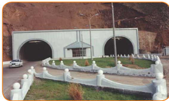
74-rasm. Qamchiq dovonidagi tunnel.
